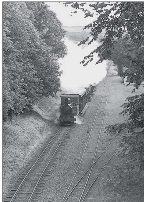
Far left: looking over the parapet of the road bridge at the south (Port Erin) end of the station on 30 May 1953, the track arrangement is clear. Note the Y point, far more common in IoMR station trackwork than left or right hand turnouts. The line to the right goes to the raised goods platform. Photo: the late David Odabashian.
