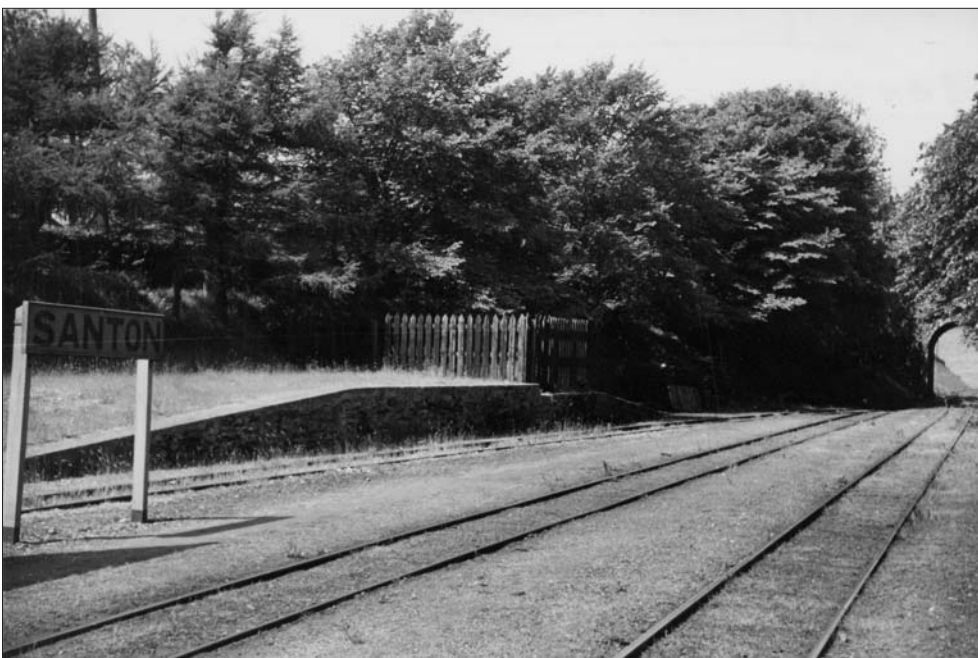
Below left: a 30 May 1953 view of the long advertising hoarding, constructed of timber panelling supported by old rails. Such screens were constructed to hide goods facilities.
